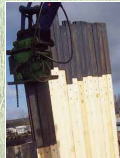
KLP® Combi-pile planking - marina 'Jachthaven Akkrum' (NL)
