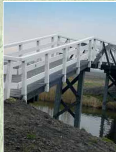
KLP® Arched suspension bridge - 'Gemeente Opmeer' (NL)
